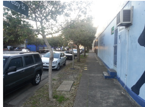
Figure 2.10: Cressy Street pedestrian paths (looking west)
